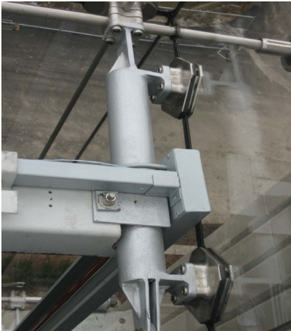
Figure 10: Horizontal cable penetration through the glass. The vertical rail below is part of the motorized blind system.
