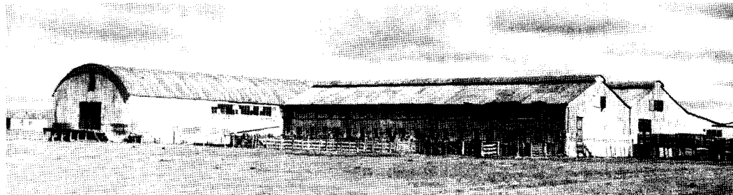
Figure 10 Shearing shed Ciaike Sheep Station, Patagonia, Chile
