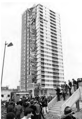
Figuur 4.1: Instorting Ronan Point, Londen, 1968.
