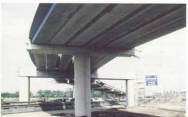
Figs. 2. Cast-in-situ bridge, extended formwork a hinder for the traffic (a) and a precast bridge a minimum of hinder for the traffic (b)
