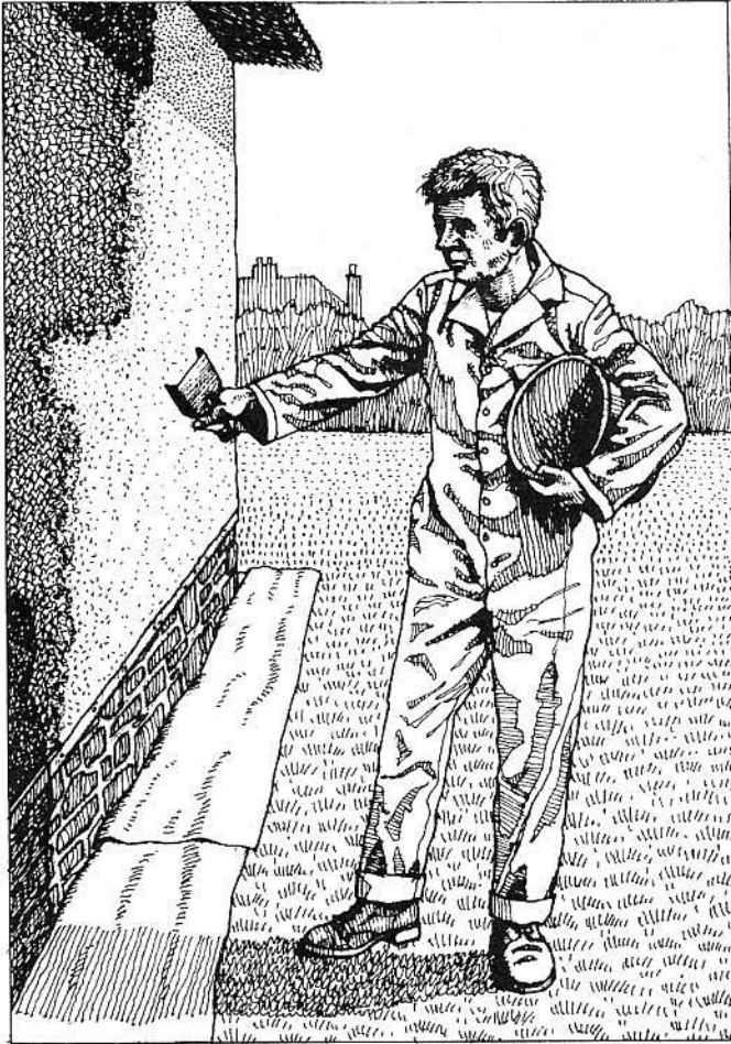
Fig. 2 Roughcasting a cob wall
