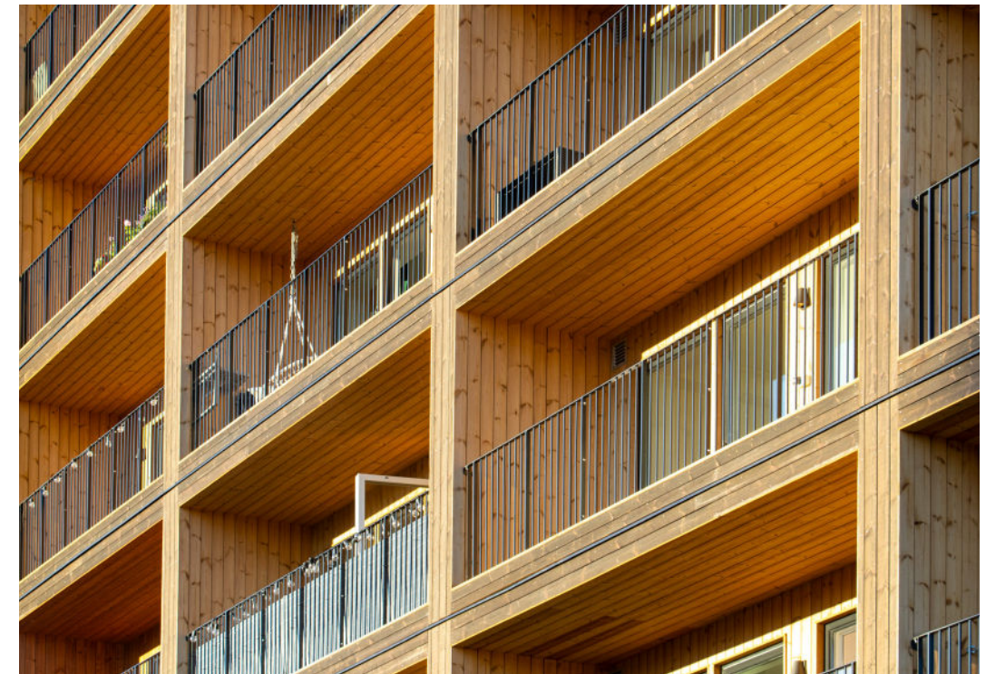
Kajstaden Tall Timber Building - CF Møller Architects (Fotograaf: Nikolaj Jakobsen)
