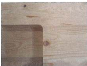
Rounded corners on VI panels
