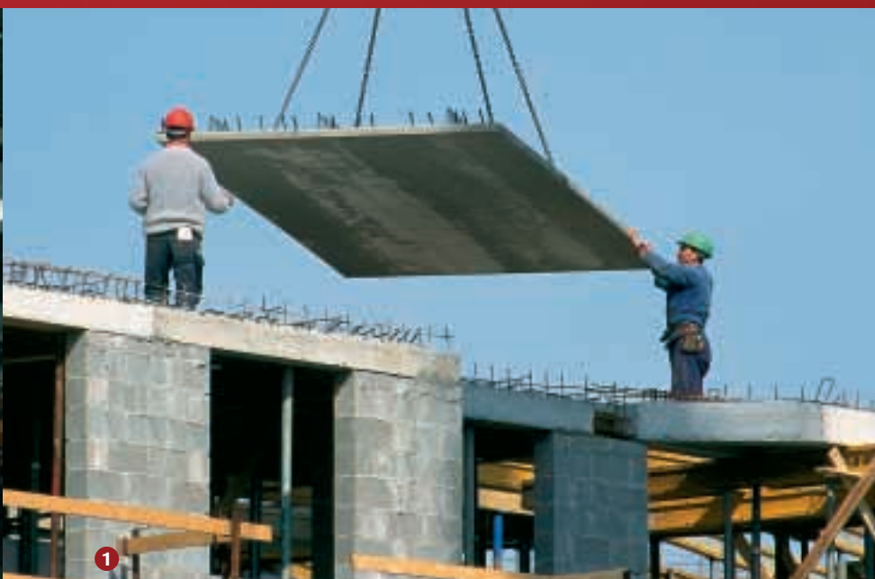
Predallen in structureel lichtbeton
