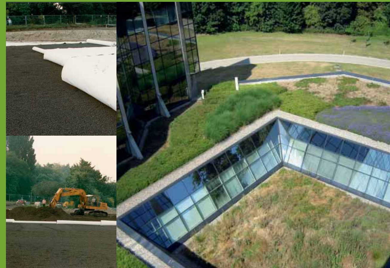
Waterloo, Office Park
