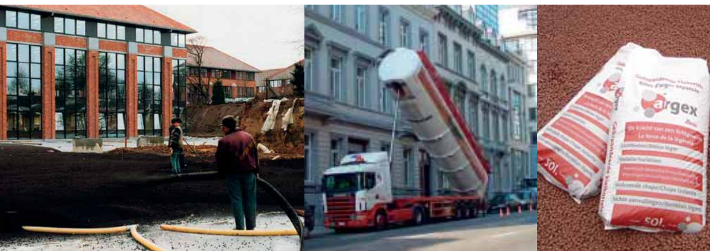
Waterloo, Office Park
