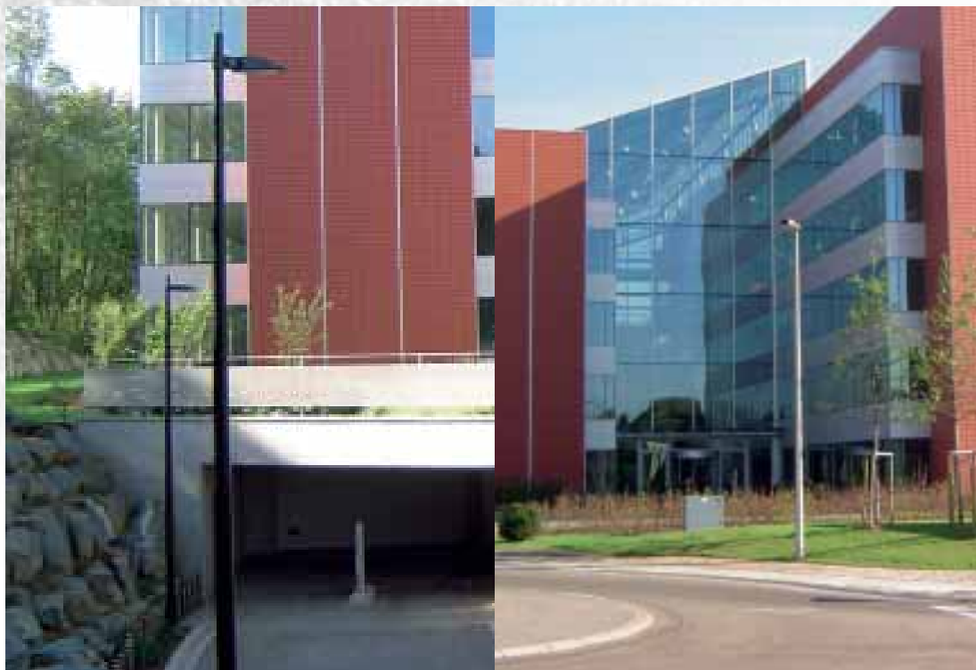
Waterloo, Office Park
