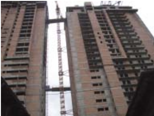
Under construction. Apartment buildings with over 20 storeys. 520 Sovent fittings installed.
