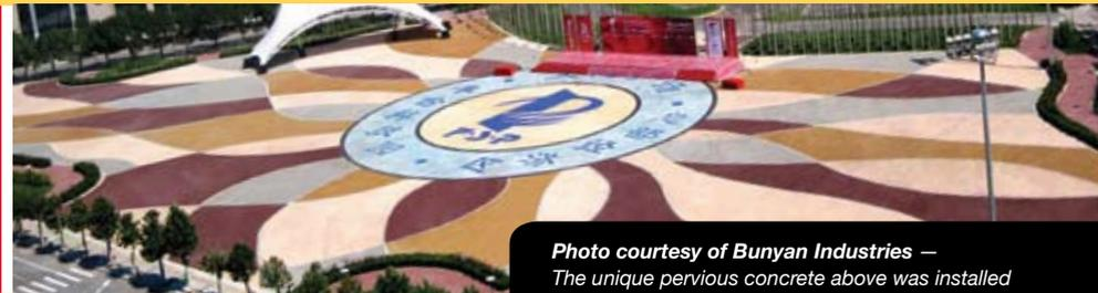
*Photo courtesy of Bunyan Industries — The unique pervious concrete above was installed for the 2008 Summer Olympics in Beijing. Stamped concrete was used to create the light blue ring that encircles the logo.*
